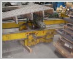
Stall Overhead Crane
