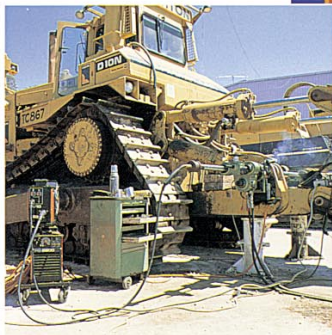
Workshop quality repairs in the field.
